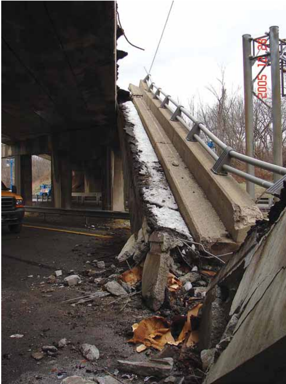
PHOTO OF COLLAPSED BOX GIRDER, BRIDGE ON I-70
