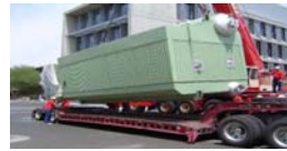
Boiler & Boiler Burner Replacement
