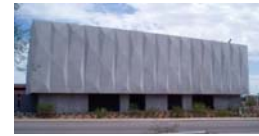
Combined Heat & Power (CHP) Plant
