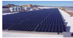
First Campus PV System (184 kW DC)
