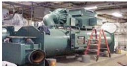
Energy & Central Plant Retrofit
