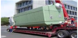
Boiler & Boiler Burner Replacement
