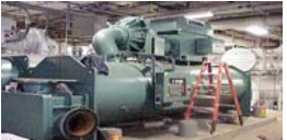
Energy & Central Plant Retrofit
