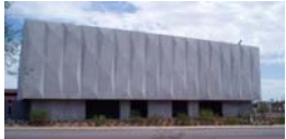
Combined Heat & Power (CHP) Plant
