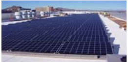
First Campus PV System (184 kW DC)
