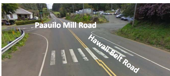
Existing faded crosswalk at Paauiilo Mill Road, looking south.
