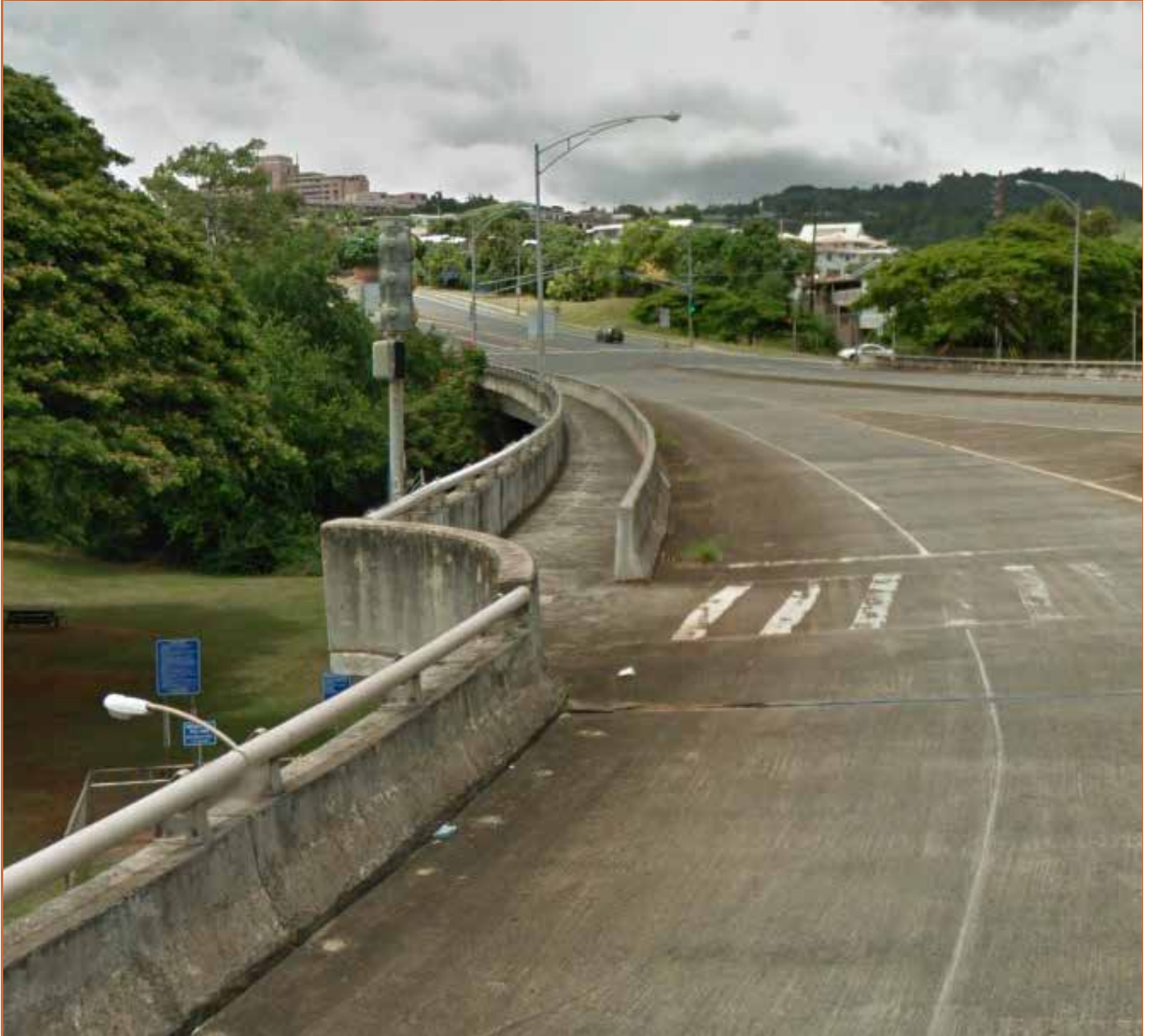
A concrete barrier along the sidewalk separates pedestrians from traffic near the Salt Lake neighborhood
