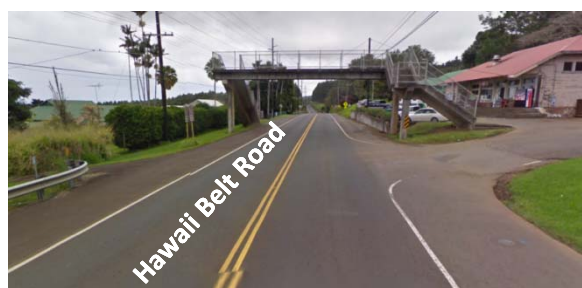
Existing pedestrian bridge, looking south
