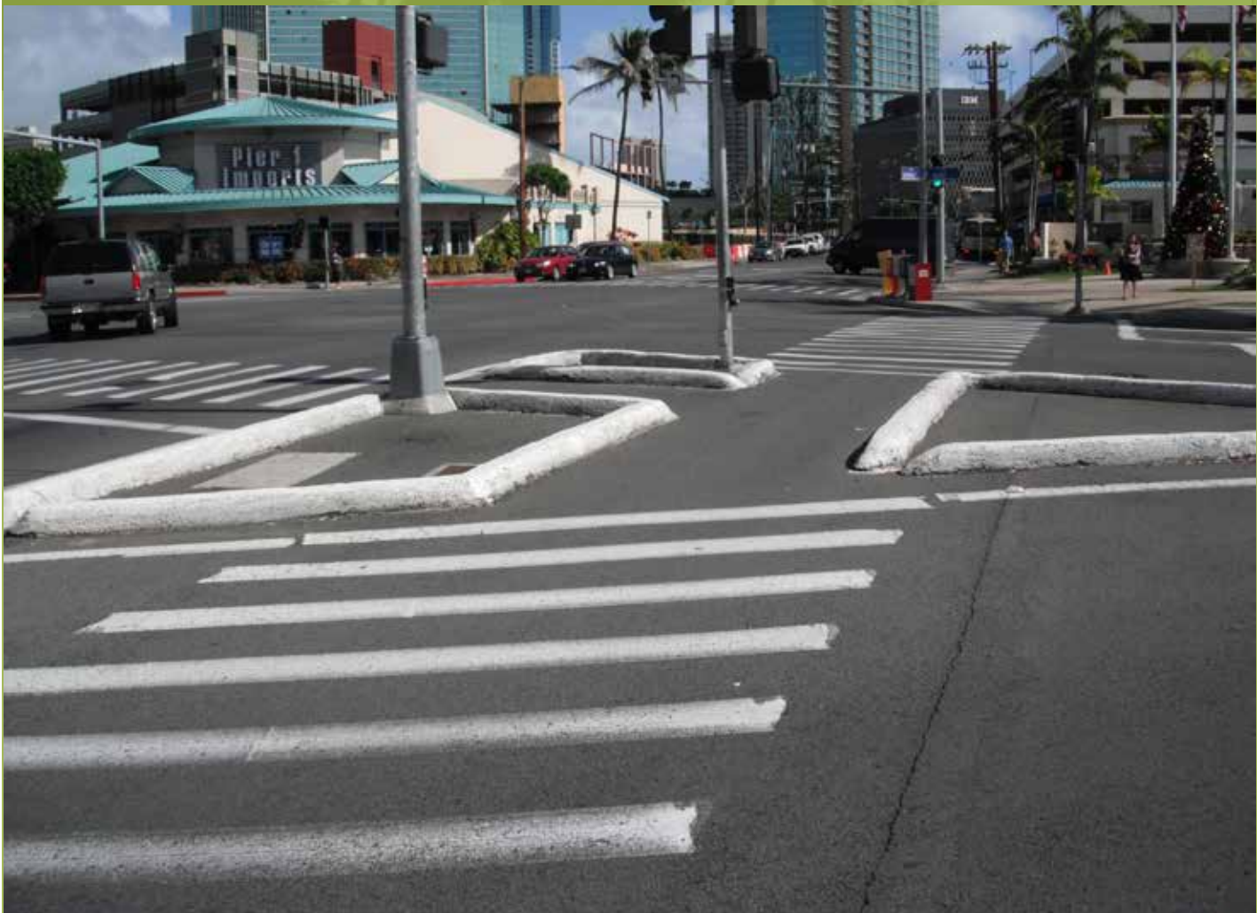
The median refuge island provides a cut-through for accessibility and shortens the crossing distance at this wide intersection in Honolulu.
