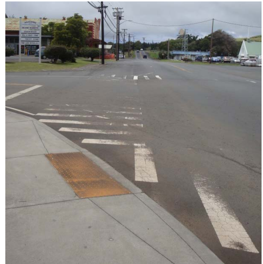
Faded crosswalks at Kalaiki Road
