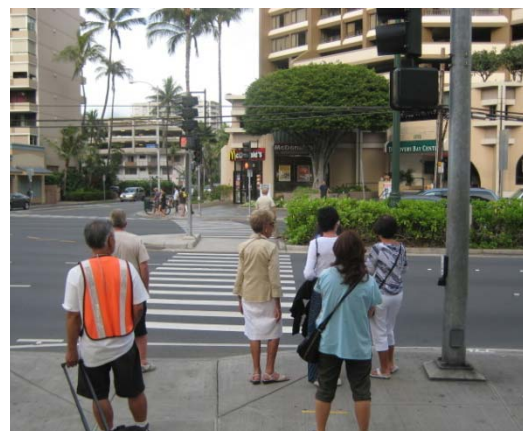
Looking northeast: Straightened crosswalk across Ala Moana Blvd at Hobron Lane.
