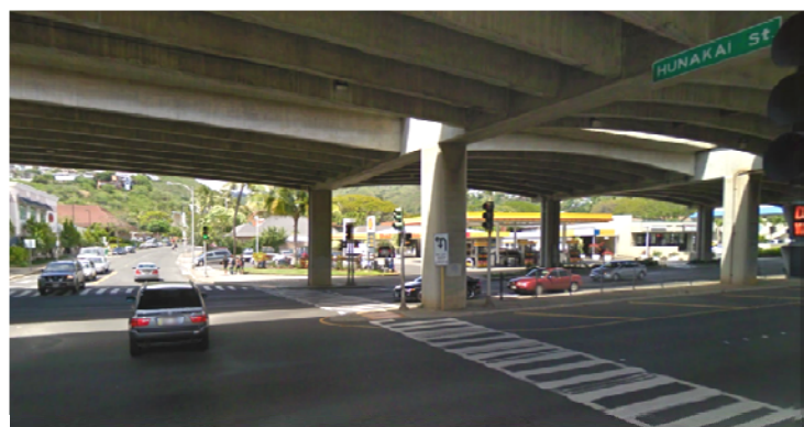
Waialae Ave. / Hunakai St. Intersection (looking mauka)
