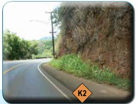
Kuhio Highway, between Wilcox Memorial Hospital and Hanamaulu Road
