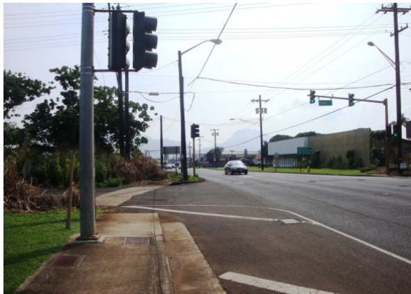
Sidewalk gap along Kuhio Highway; looking southbound
