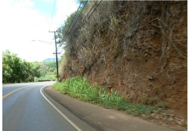
Kuhio Highway heading east; Existing 2-3' sidewalk on the makai side
