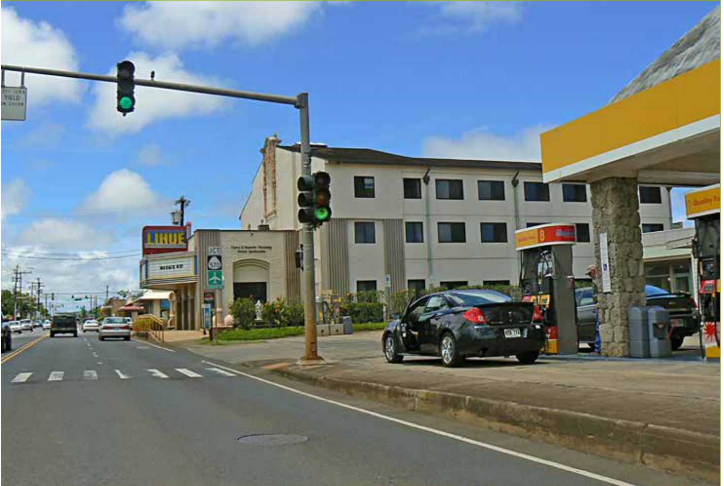
Roadway and pedestrian facilities along Kuhio Highway in Lihue, Kauai
