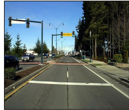
Figure 30: Advance Stop/Yield Lines
