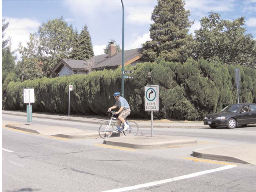
Cyclist on a “Bikeway” (a.k.a., bicycle boulevard) in Vancouver, British Columbia, Canada, illustrating a vehicle traffic diverter, bike cut-through, and arterial-crossing bicycle and pedestrian refuges
