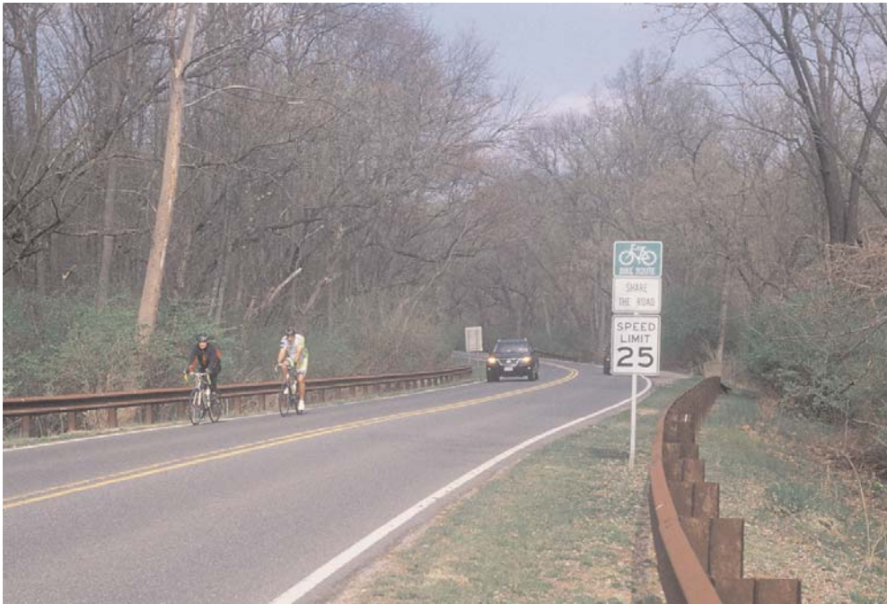
In Montgomery County, MD, the on-road bike route, which parallels the trail (bottom) sees mostly avid cyclists
