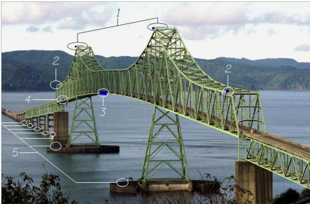
**Figure 6: Locations of the five different types of solar lights on the Astoria-Megler Bridge**
