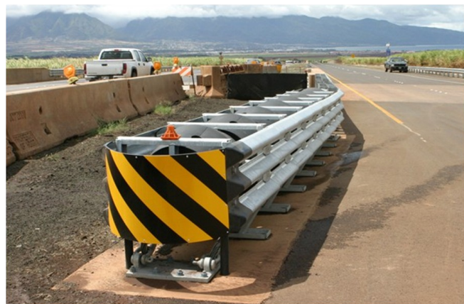
Guardrail on the Haleakala Highway improved with energy-absorbing crash attenuator. Image: Hawaii Department of Transportation.
