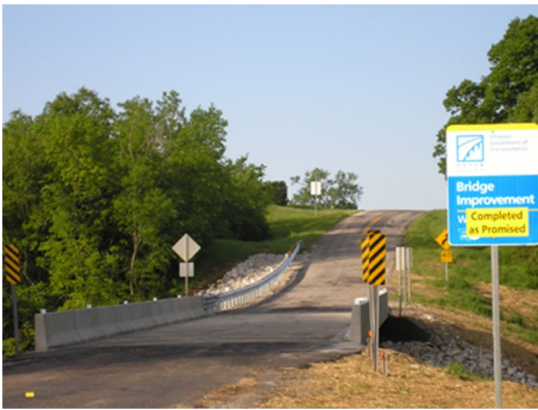
Henry County, Route N over Honey Creek, part of Missouri's Safe and Sound bridge improvement project. Image: Missouri Department of Transportation.
