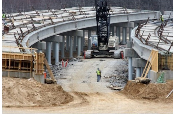
Work on the final segment of the Tenn. 85 outer loop highway around Memphis, Tennessee. Image: The Commercial Appeal.
