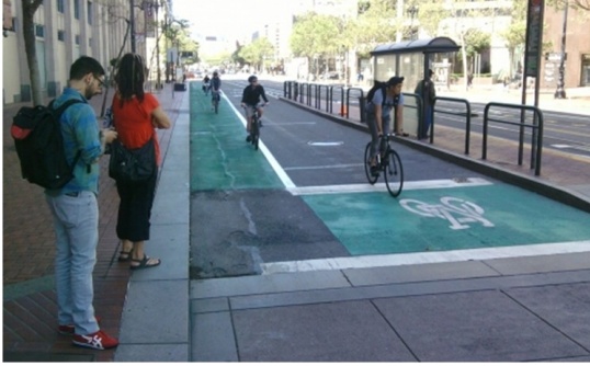
Green bike lane and bike box along San Francisco's Market Street. Image: L.A. Eco-Village Blog.
