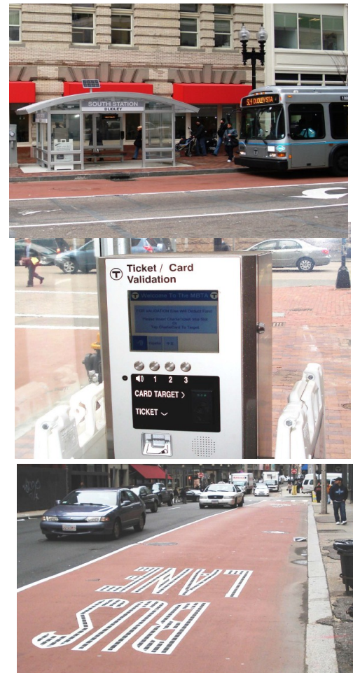
Silver line, Washington Street: station, off-board ticket /card validation system and painted bus lane
