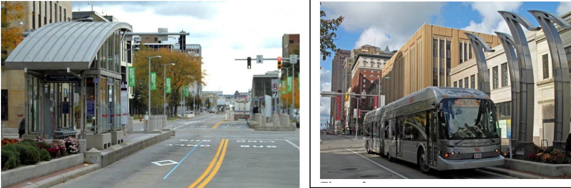
Station design; articulated bus next to sculpture pieces along the HealthLine BRT corridor in Cleveland
