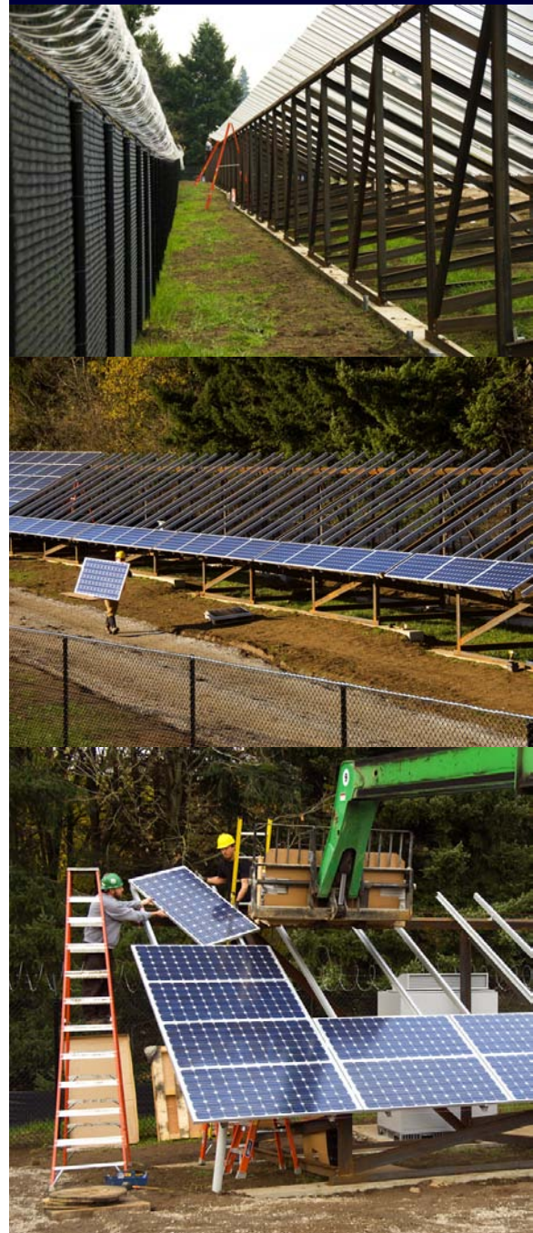
Installation of the steel racking system, aluminum framing and solar PV modules.
