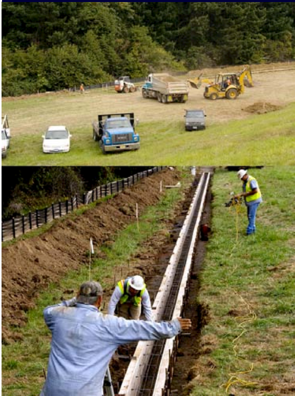
Installation of the security fence.
