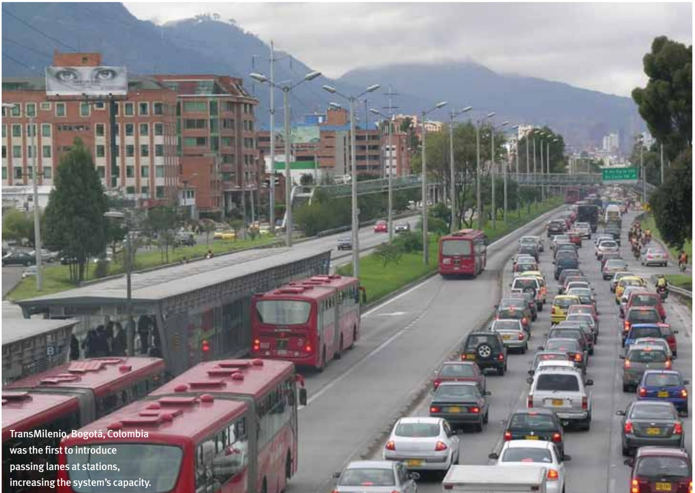
TransMilenio, Bogotá, Colombia was the first to introduce passing lanes at stations, increasing the system's capacity.
