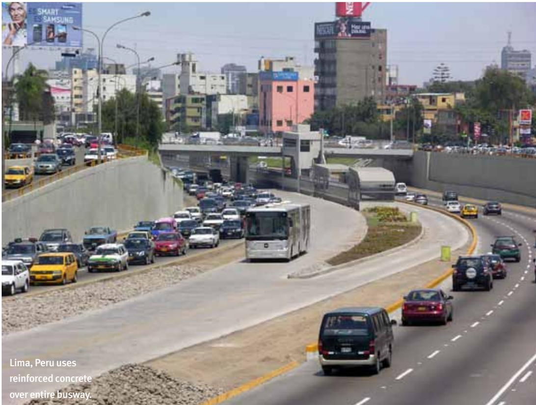
Lima, Peru uses reinforced concrete over entire busway.
