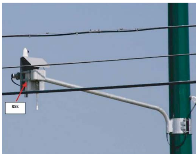
Figure 22. Typical RSE installation.
